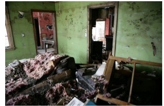
SNI PER was used to clean-up mold and disinfect after Katrina
